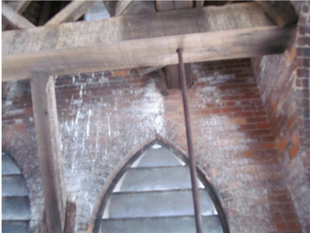
Main wood structural support beam with steel tension rod. Structural wood beams are pocketed into the brick structure.
